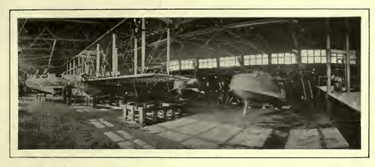
THE CURTISS ABROPLANE FACTORY: AN ABROPLANE APPROACHING COMPLETION, AND "BOATS" AWAITING THEIR WINGS.
