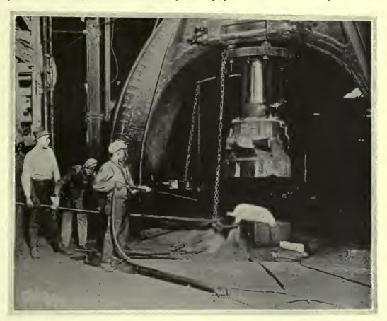
FORGING A 14-INCH SHELL BY STEAM HAMMER.
